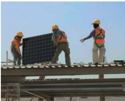
Enviromena's technical team at work on site
